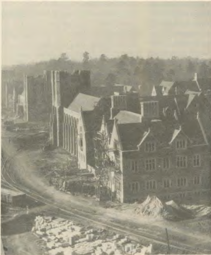
The Old Law School Building under construction
